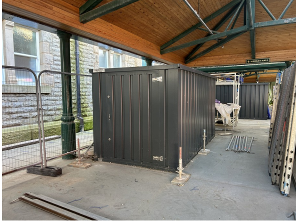
Typical storage cabin under the rear pavilion - surrounding scaffolding, fencing and site materials are excluded
