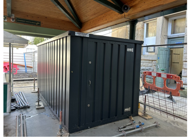
Typical storage cabin and current access setting - all surrounding temporary works and site equipment are excluded
