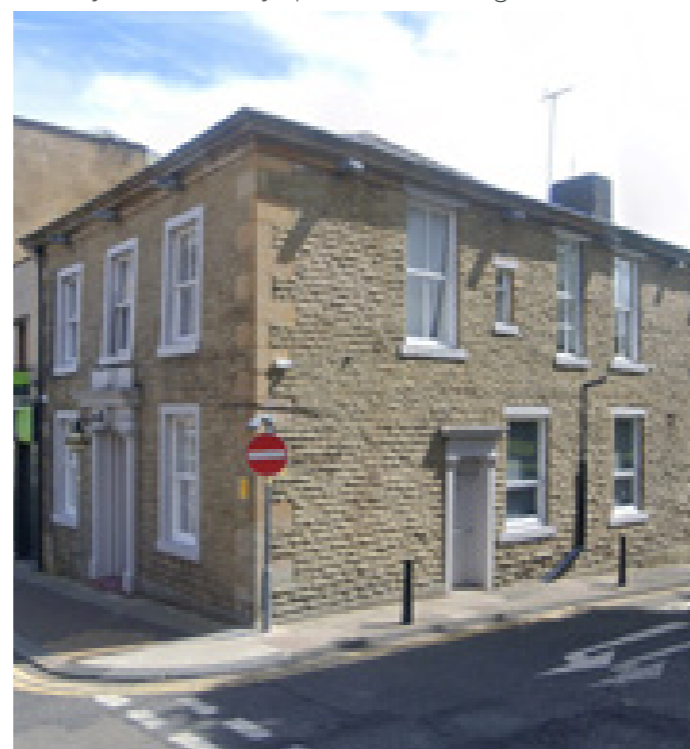
4 - Former Bees Knees Public House, St James Street- Approved Change of use of former public house to 13 apartments.
