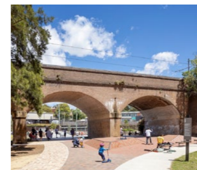
Example of parkland place spaces under a railway viaduct
