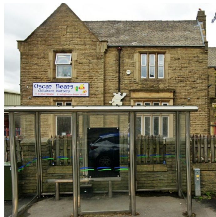
1 - Parsonage House, Blackburn Road- Granted Planning Permission. Conversion of a 2 storey and basement nursery into a 4 storey apartment building.
